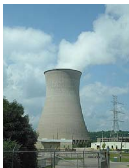
William H. Zimmer Power Plant, Moscow, OH
